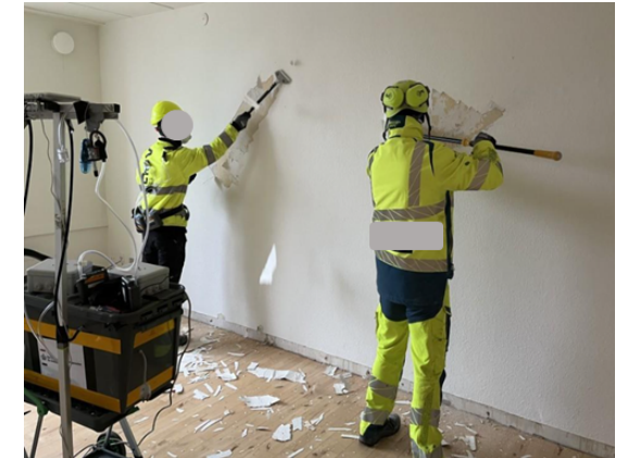
Building renovation or demolition
